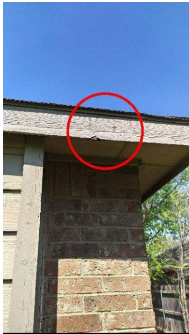
Damaged soffit
