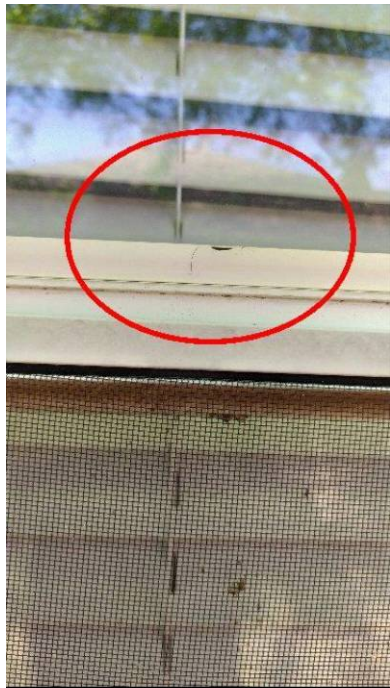
Damaged bead
