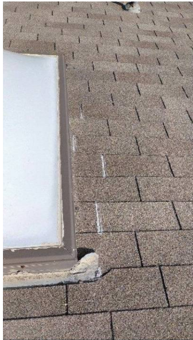
Sealant repair
